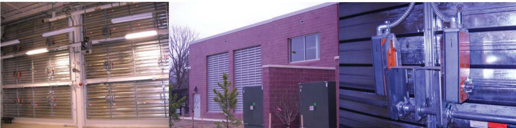
generator plant at Fort Belvoir Hospital, which must be able to deliver full power to the hospital in just 6 seconds. Make-up air is required for the hospital generators to leap into action, which means the dampers must open rapidly to instantaneously deliver up to 100,000 CFM to each of the two generators per room in the plant. Given the challenging application, Cummings was hesitant to use standard methodology.
